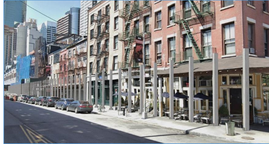
12-ft high posts to hold stop logs
